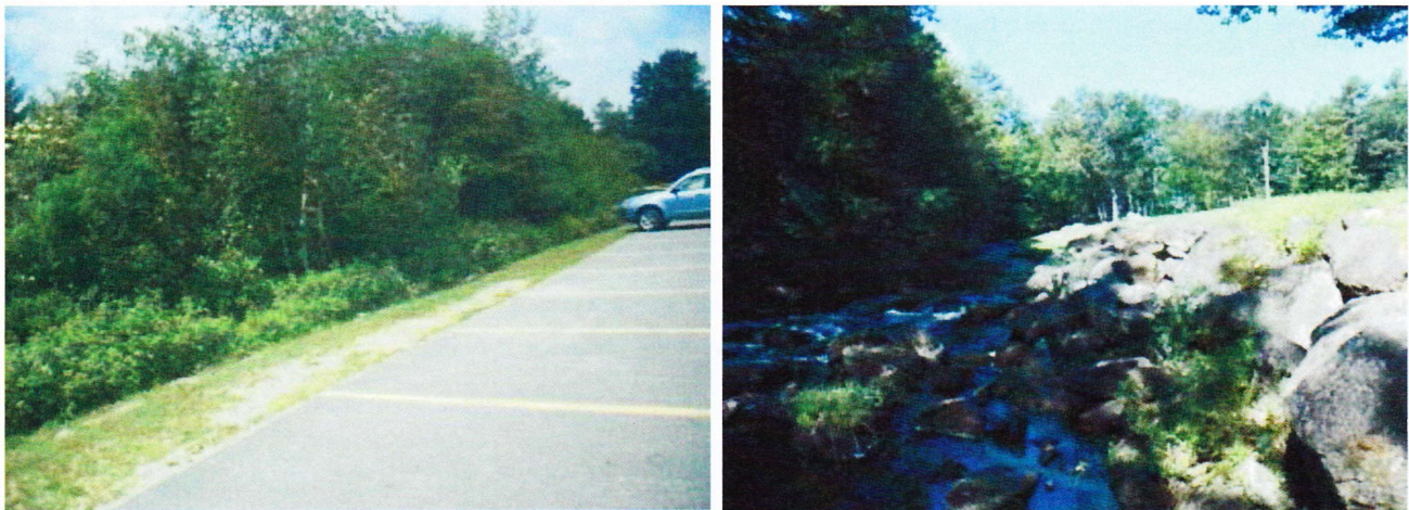
Locations along an unnamed wild brook trout stream (left) and the Lane River (right), both in Sutton where riparian areas have been removed. The natural stream bank stability, filtering ability and shading of a stream has been reduced. Boulders have been placed overtime along this location of the Lane River to prevent damage to the adjacent field.
