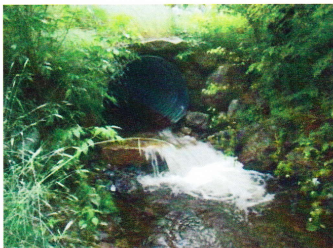
Examples of undersized culverts on Kings Brook at Poor Farm Rd in Sutton (left) and an unnamed stream at Basin Hill Rd in Warner (right). Crossings not designed with the accommodation of fish passage and sediment conveyance make it difficult for fish to access more desirable habitats, increase erosion and sedimentation rates, and have an increased likelihood of failing.
