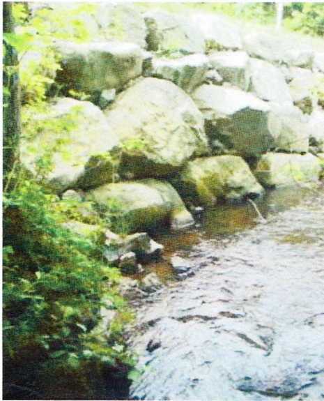
Examples of shoreline bank armoring on Bartlett Brook in Warner (left) and Lion Brook (New London). During high flows, the stream is precluded from accessing its floodplain where the velocity of flows could be naturally reduced. Instead, erosive flows continue to downstream areas.
